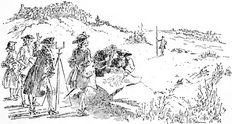
SURVEYORS LAYING OUT BALTIMORE
